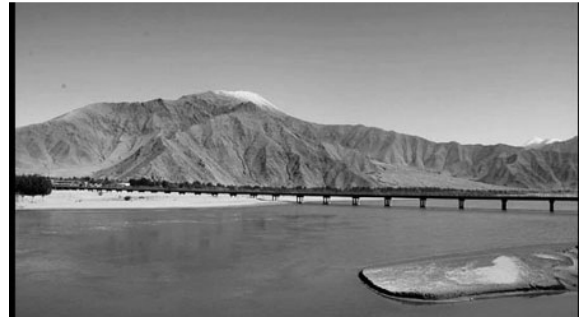
Fig. 2 Photograph showing the redundancy of the bridge due to changing course of the river
